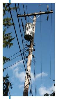
Power flows through a transformer drum on a power pole into a kilowatt-hour meter. The meter measures the amount of energy going into the home so
